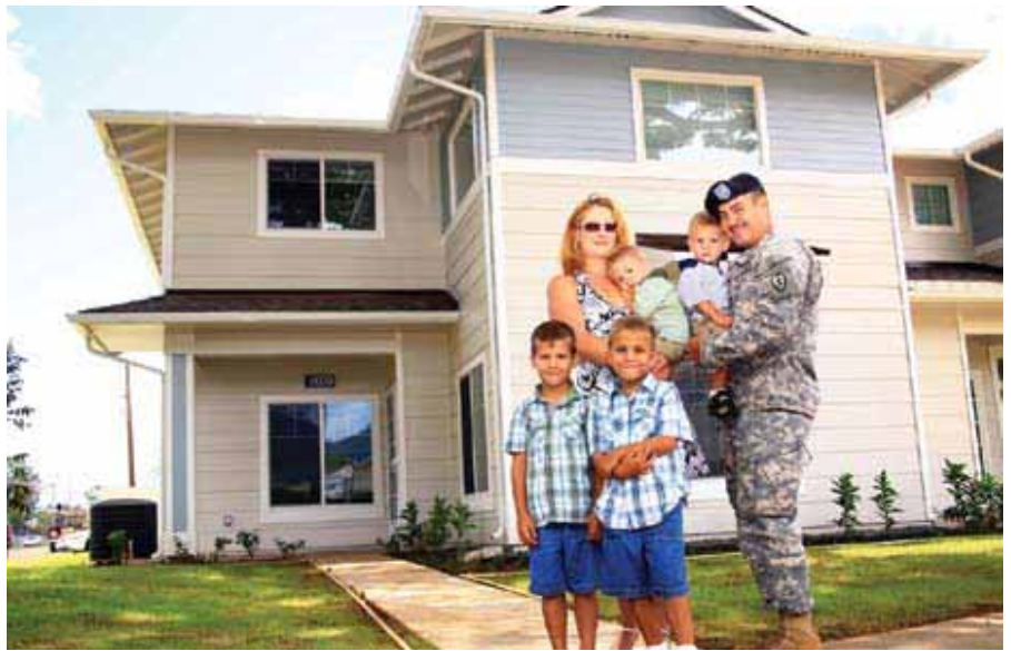
This home developed by Actus Lend Lease in the Kaena neighborhood at Schofield Barracks is one of the first four LEED gold-certified homes on Oahu and the first LEED gold homes on a U.S. military installation.
