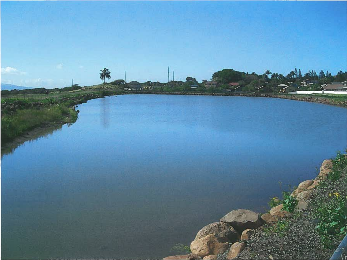
Reservoir 6 Waikapu Stream
