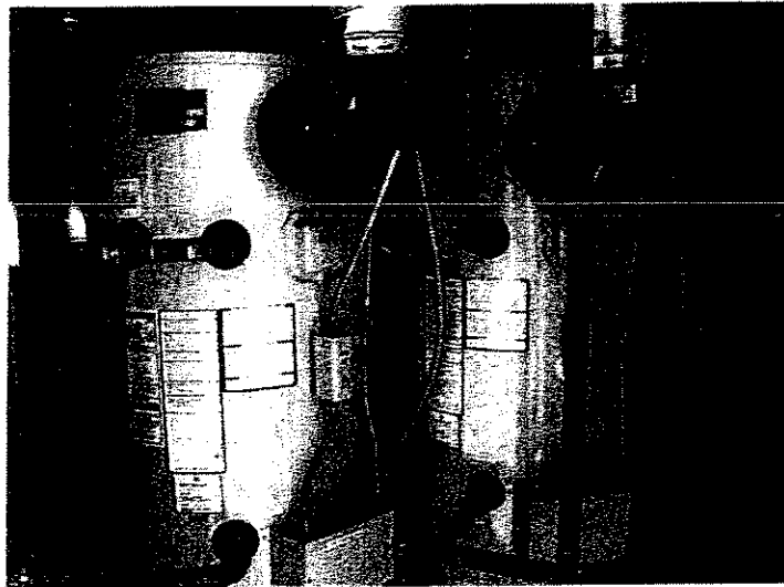
Hot Water Heaters
