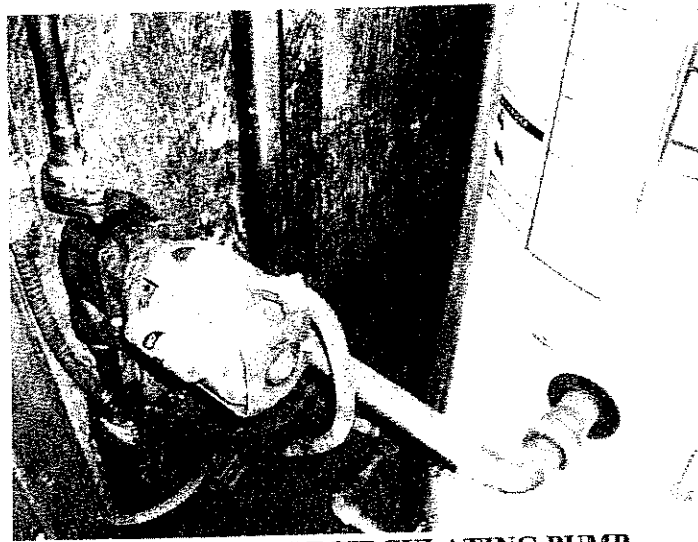
HOT WATER RECIRCULATING PUMP
