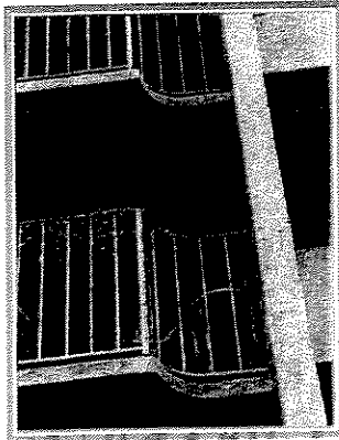
Photos 6 & 7: Showing concrete spall at apartment lanai edge.
