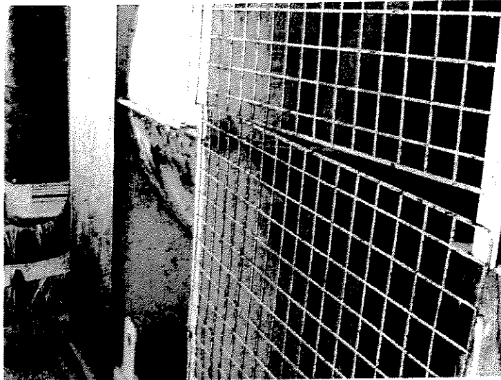
Cooling Tower Fan in Poor Condition
